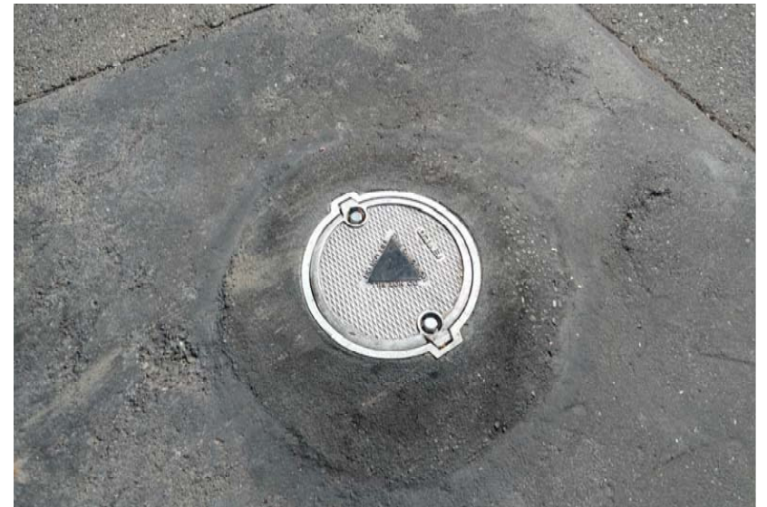
Monitoring well located east of the Subject Property
