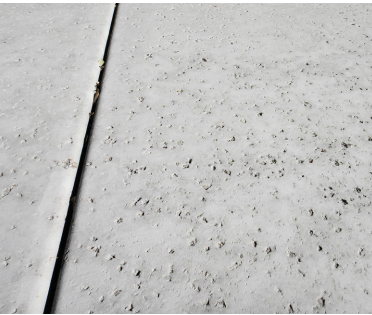
CONCRETE PAD WITH SALT FINISH
