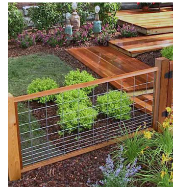
4 railing framed hog wire 2x4" maximum openings
