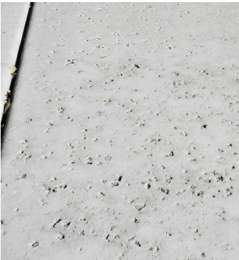
5 parklet surface concrete pad with salt finish
