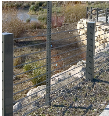
4 railing tensioned cable railing 3.5" maximum spacing
