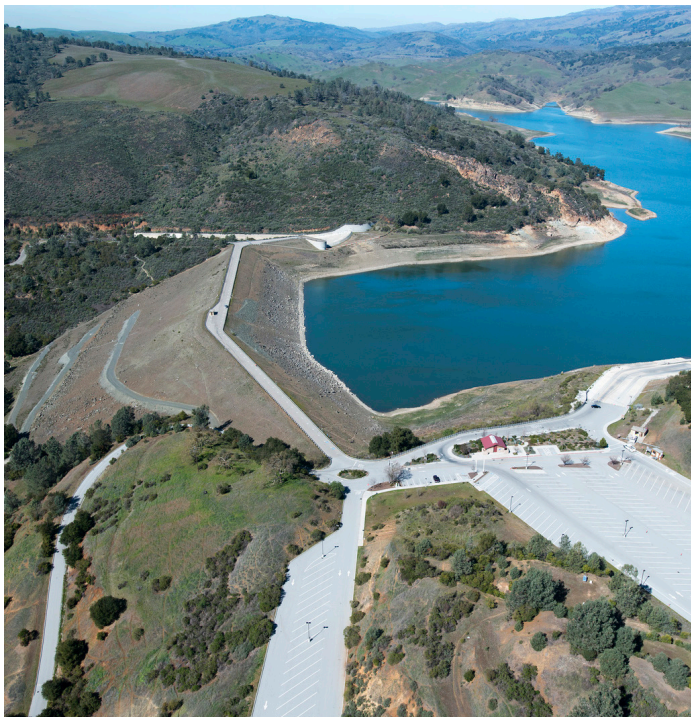
Aerial view of Anderson Dam
