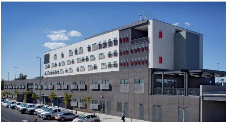
SMUD Office & Operations Building, Sacramento
