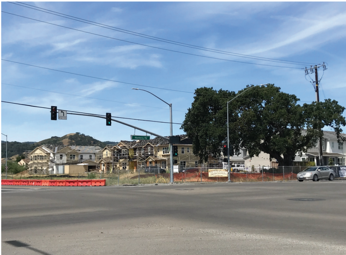
Photo 3: View of the two-story townhomes being constructed on the corner of Monterey Road and Butterfield Blvd looking northwest.
