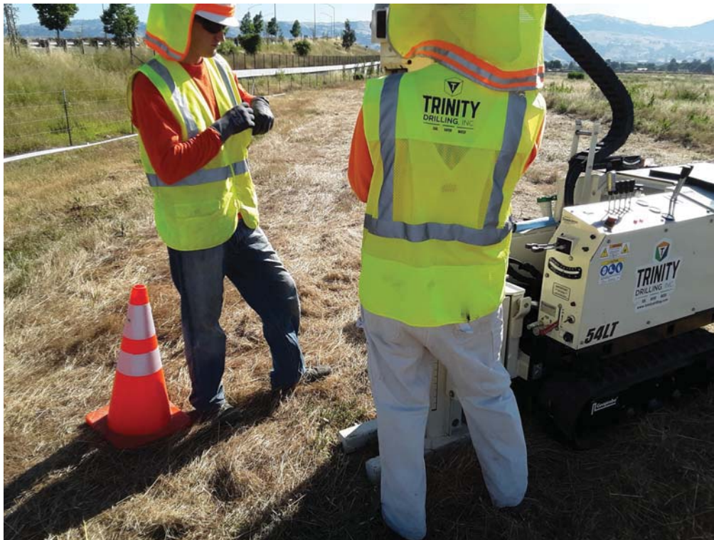
Track rig was used due to the limited access to the Site
