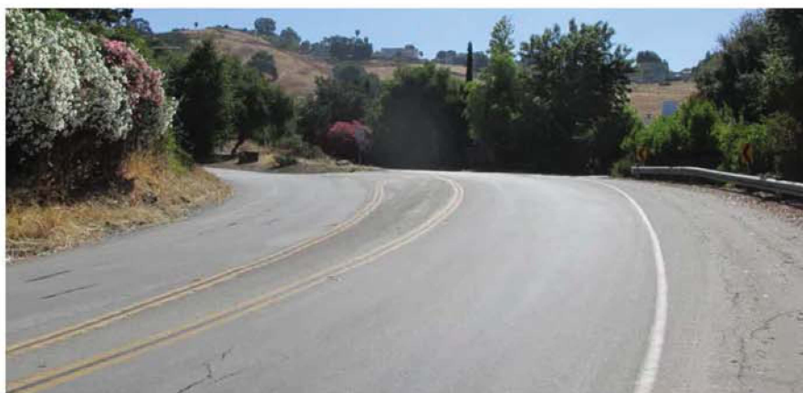
Photo 19. Road shoulders cleared as fuel breaks.
