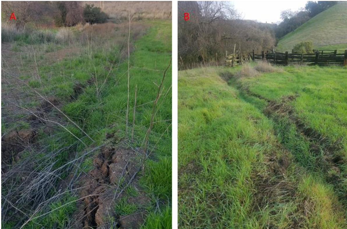
Figure 5. Photos taken of subsidence fissures forming in areas of fault localization trenching (location indicated in Figure 1). This subsidence occurred during the rain storm in early January, 2019. The fissures extend been 50 and 200 feet, are not limited to excavation location (i.e., extend beyond area of trenching) and are between 1-3 feet deep and 3-4 feet across.
