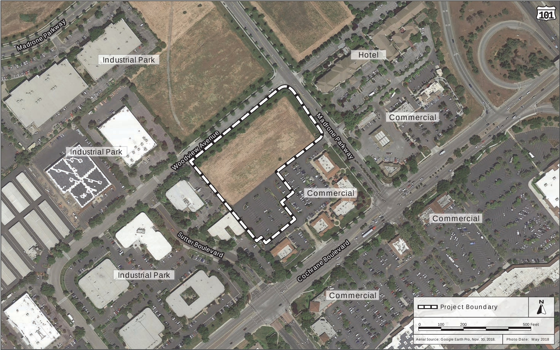
AERIAL PHOTOGRAPH AND SURROUNDING LAND USES
