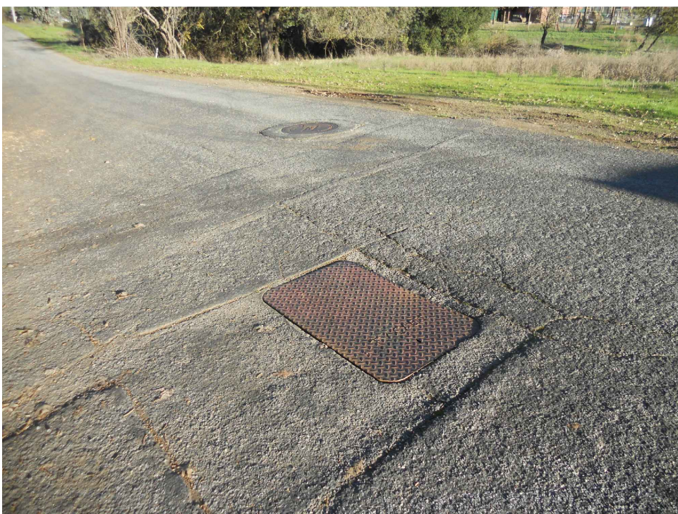
TYPICAL CONDITION OF SABINI COURT.
