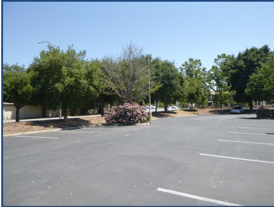
Portion of Community Center parking lot to be included in project
