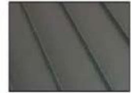
Standing Seam Metal Roofing
