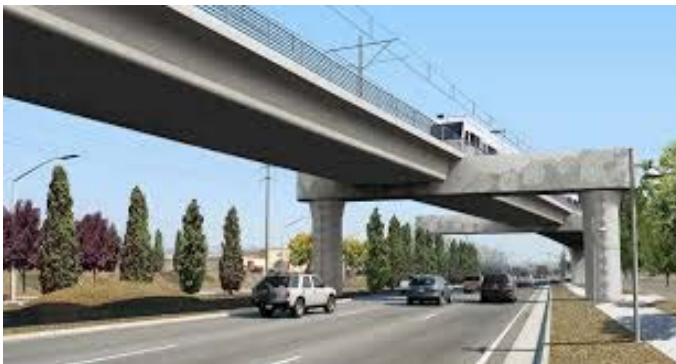
Figure 3: Straddle Bent
