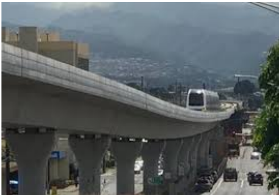
Figure 1: Railroad Viaduct on Median Source Google Images
