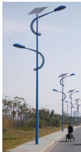
Figure 2-17: Contemporary design of a combined roadway and pedestrian-scale light fixture
