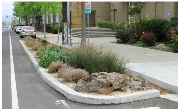
Figure 2-19: Example of planted bulb-out between parking spaces
