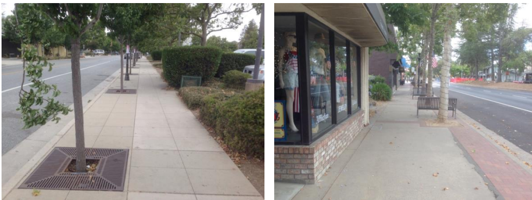
Figure 1-31: Sidewalks in the Morgan Hill Station Area
