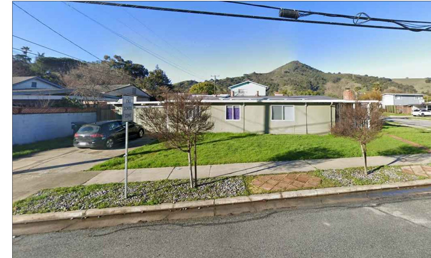
8 - NEARBY PROPERTY: 410 FARALLON DR- 1 STORY HOUSE SCALE: N/A
