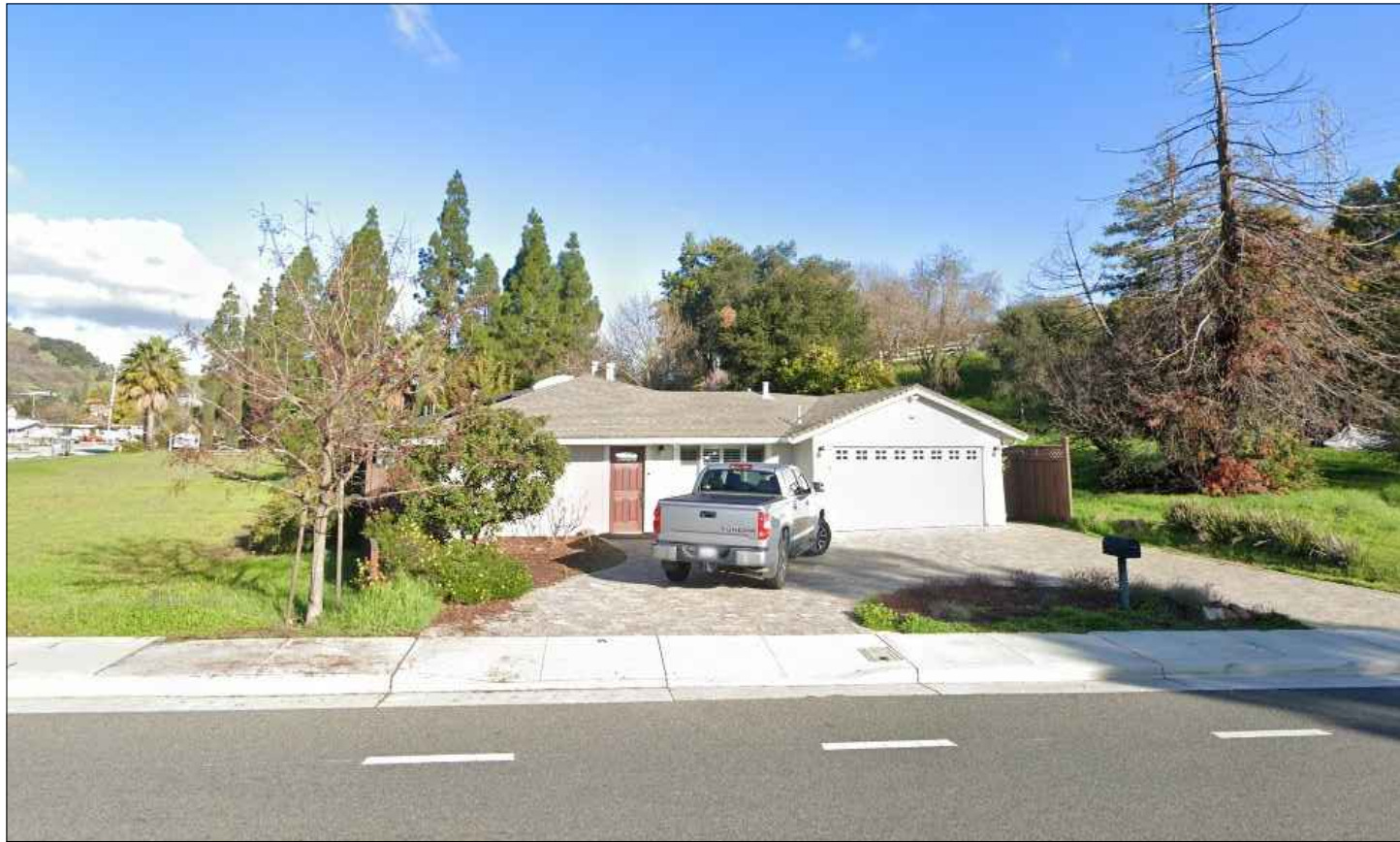
NEARBY PROPERTY: 385 W DUNNE AVE- 1 STORY HOUSE SCALE: N/A
