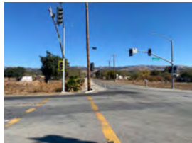
Missing or lack of sidewalks
