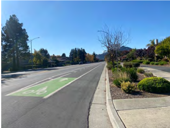
FIGURE 53 Class II Buffered bike lane on Main Ave, Morgan Hill (Source: Toole Design)
