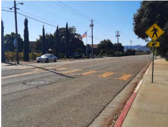
FIGURE 46 Midblock crosswalk in front of Live Oak High School, Morgan Hill (Source: Toole Design)
