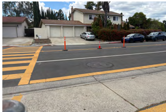
FIGURE 39 Vehicles parked along red curbs near crosswalk on La Crosse Drive
