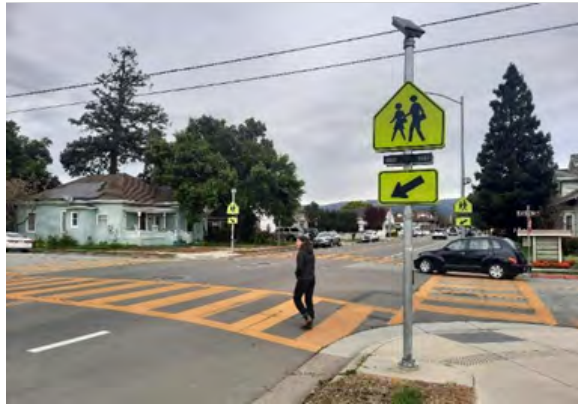
FIGURE 49 RRFB at Main Ave and Del Monte Ave, Morgan Hill (Source: Toole Design)
