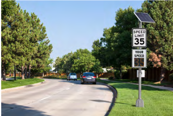
FIGURE 52 Pole-mounted Radar-Speed Sign (Source: Tim Magee)
