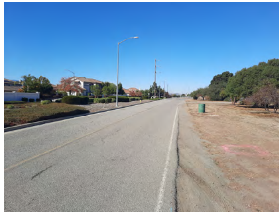
FIGURE 21 Missing sidewalks along Peet Road
