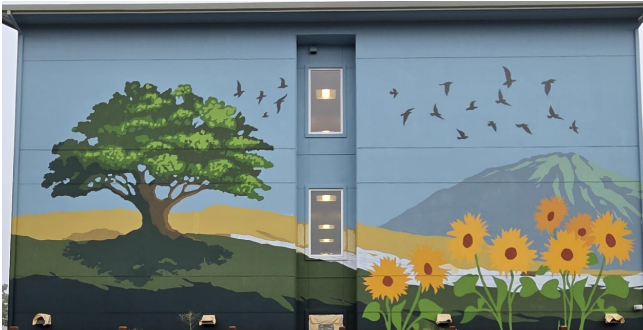
Figure 1. Mural on the Southern Facing Wall Morgan Hill Senior Housing
