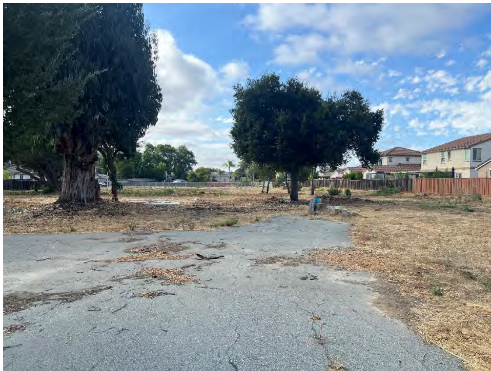
Photograph 3: View of the asphalt driveway and location of the former residential building.
