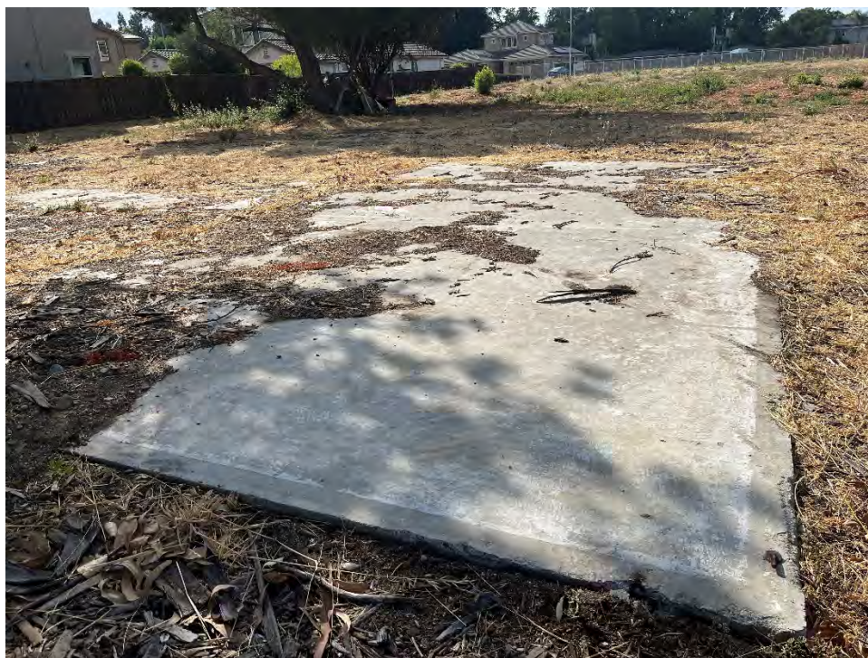
Photograph 12: Alternative view of the foundation of the former residential building.
