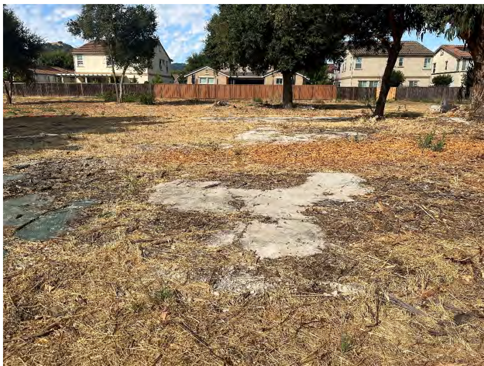
Photograph 4: View of concrete slab foundation of former building.
