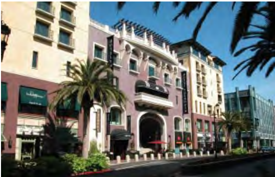
Examples of buildings with appropriate articulation.
