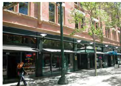
Appropriate storefront windows.
