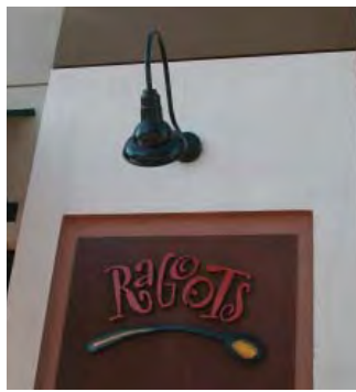
Example of sign with direct illumination.
