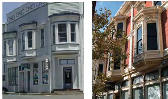
Examples of bay windows on mixed-use buildings.
