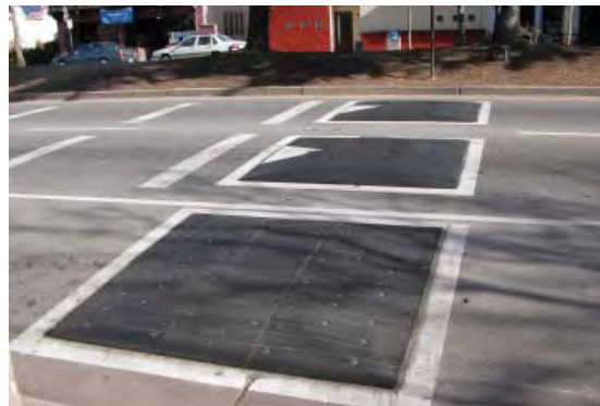
Existing speed humps on Monterey Road
