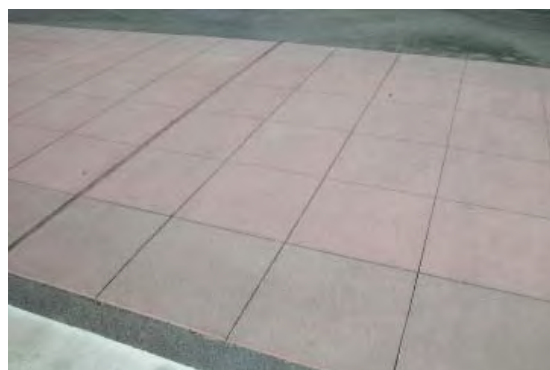
Existing special paving on Depot Street
