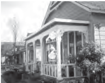
Residences converted to interesting shops and offices
