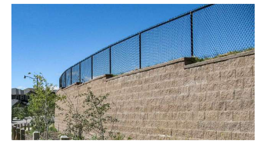
NEW CHAIN LINK FENCE ATOP NEW MODULAR MASONRY RETAINING WALL AT PROPERTY LINE WITH JACKSON SCHOOL
