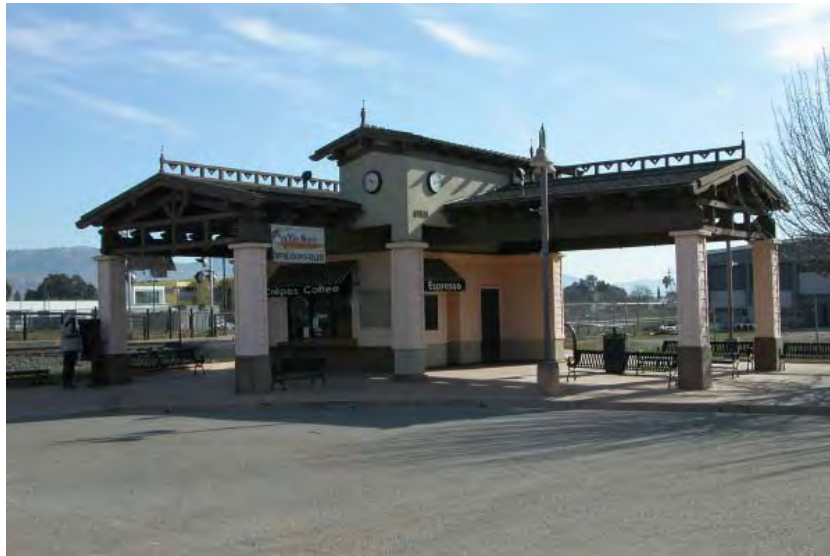
Morgan Hill Caltrain Station near Third and Depot Streets
