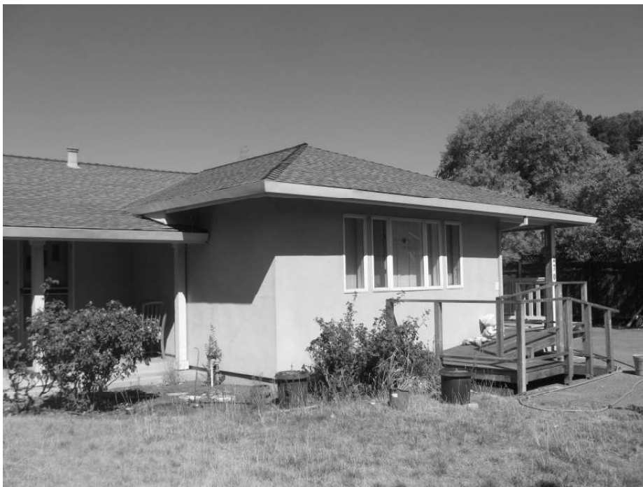
Photo 2: View of the front facade from the southeast.
