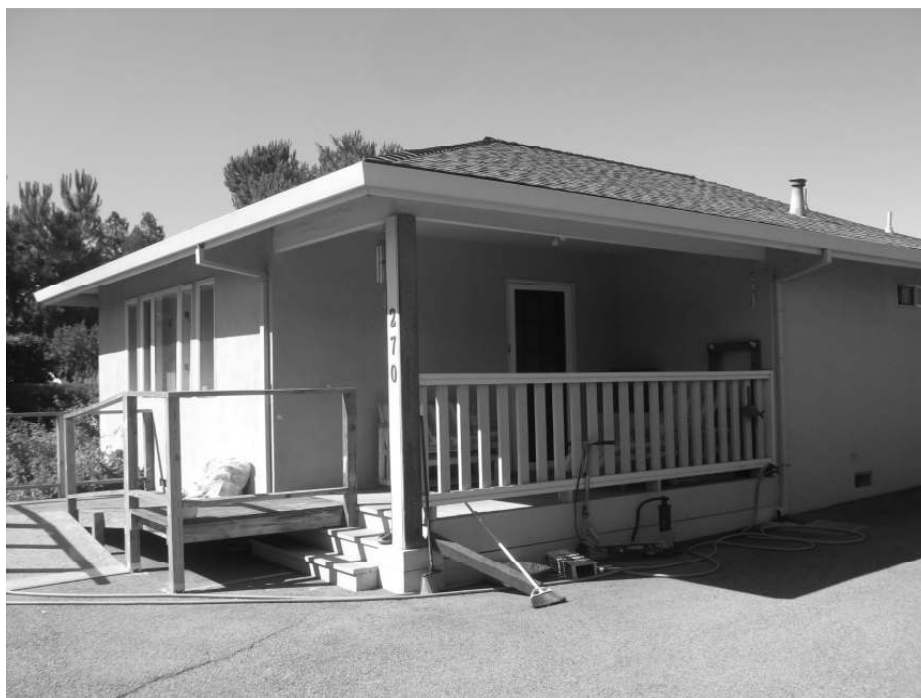
Photo 6: Oblique view of the newer corner entry.
