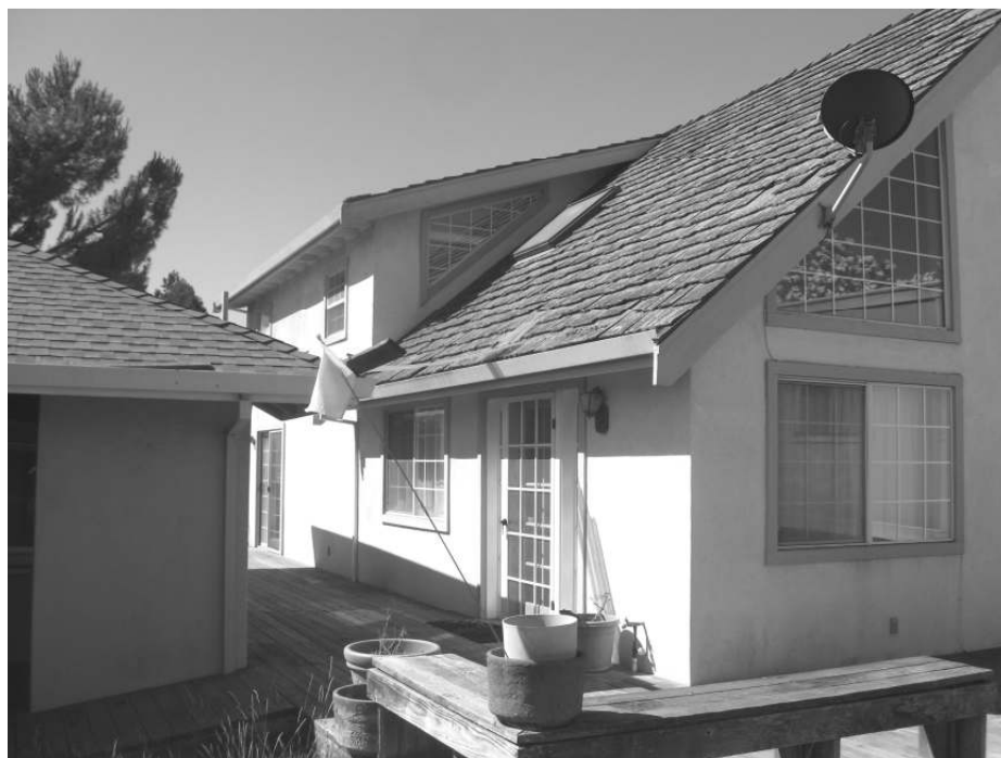
Photo 21: View along the eastern wall of the secondary residence.
