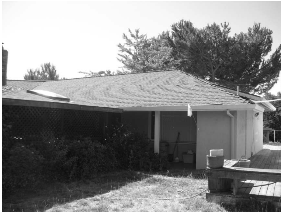
Photo 11: View of the rear portion of the residence.
