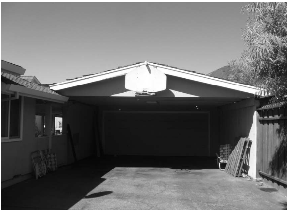
Photo 8: View of the covered carport connecting the residence and garage.
