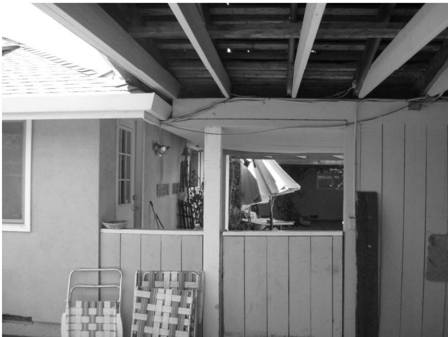
Photo 16: Detail of gate connecting the residence and garage.
