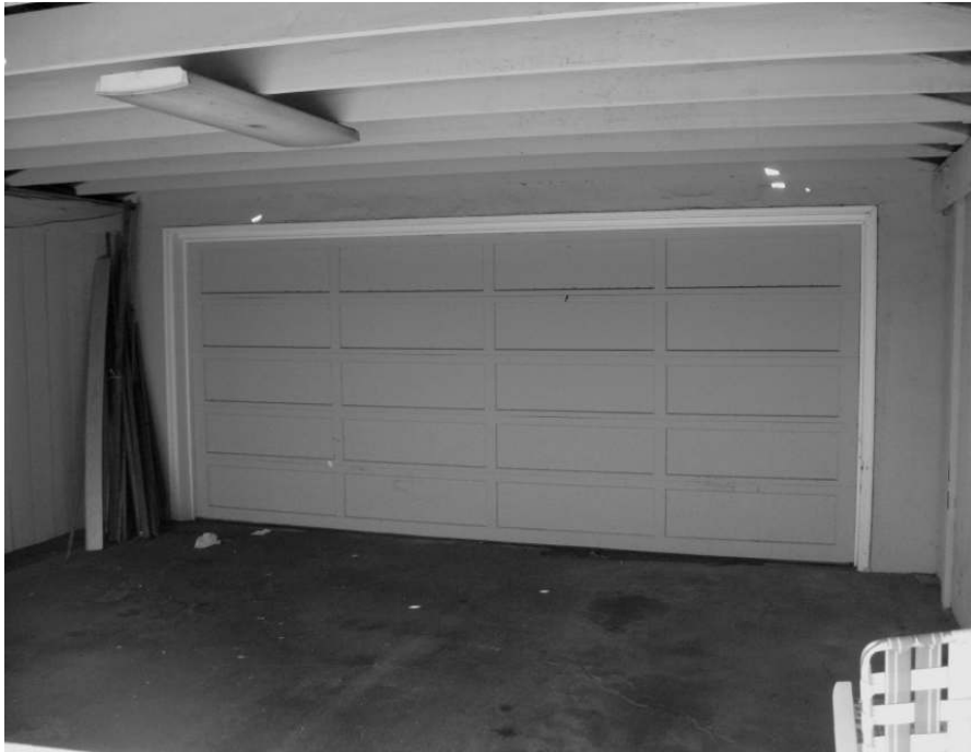
Photo 15: View of garage door beneath covered carport.
