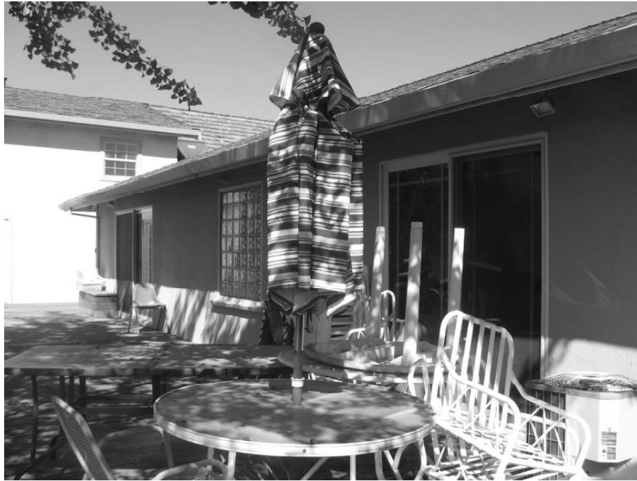
Photo 13: View of the southern facade along southern patio.
