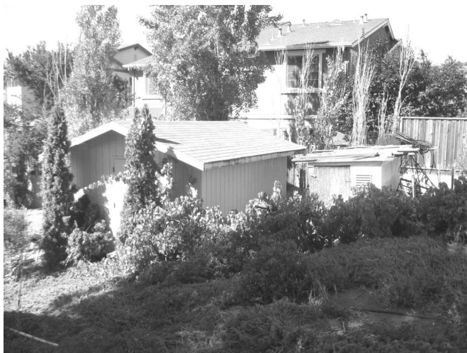
Photo 23: View of storage shed and adjacent utility shed.
