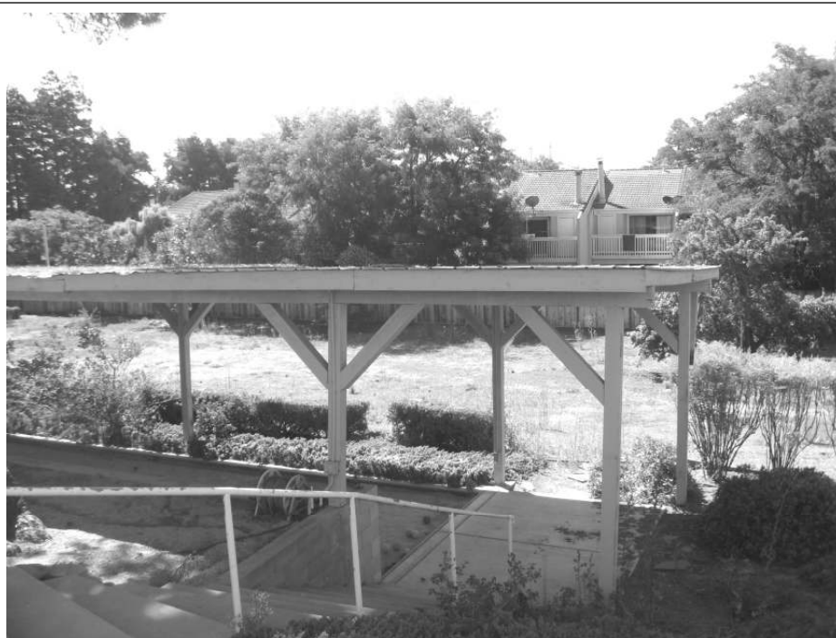
Photo 25: View of the covered bocce ball court from the patio.
