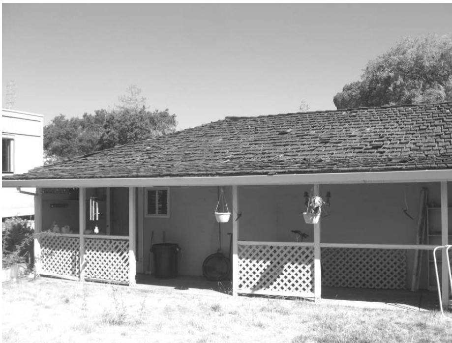
Photo 18: View of rear portion of the garage.
