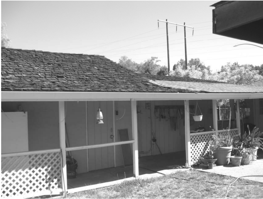
Photo 17: View of the garage with attached living space.
