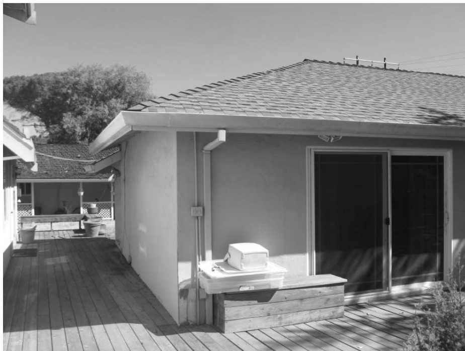
Photo 12: oblique view of the southwest corner of the residence.
