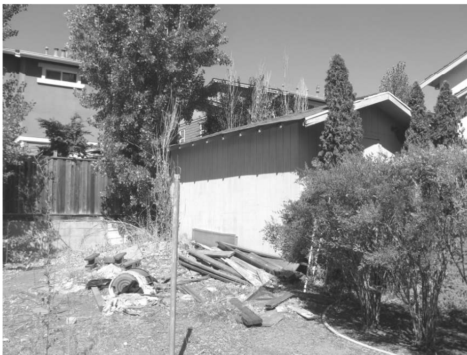
Photo 24: View of the southern side of the storage shed.
