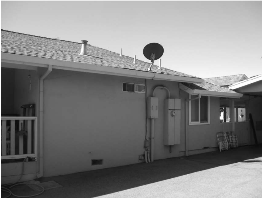
Photo 7: View along the northern facade of the residence.
