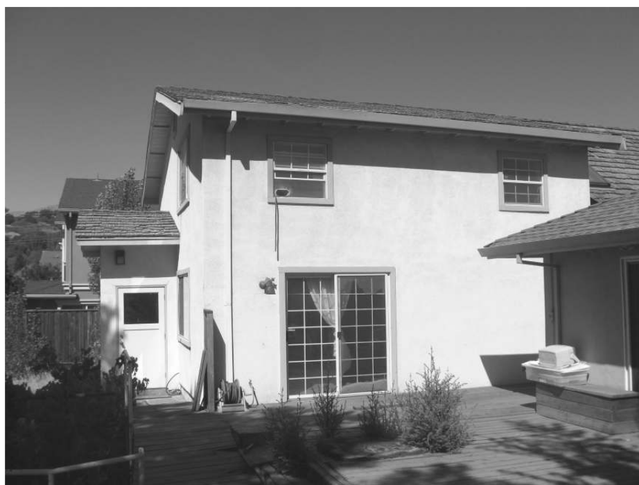
Photo 22: View of the eastern facade of the secondary residence.
