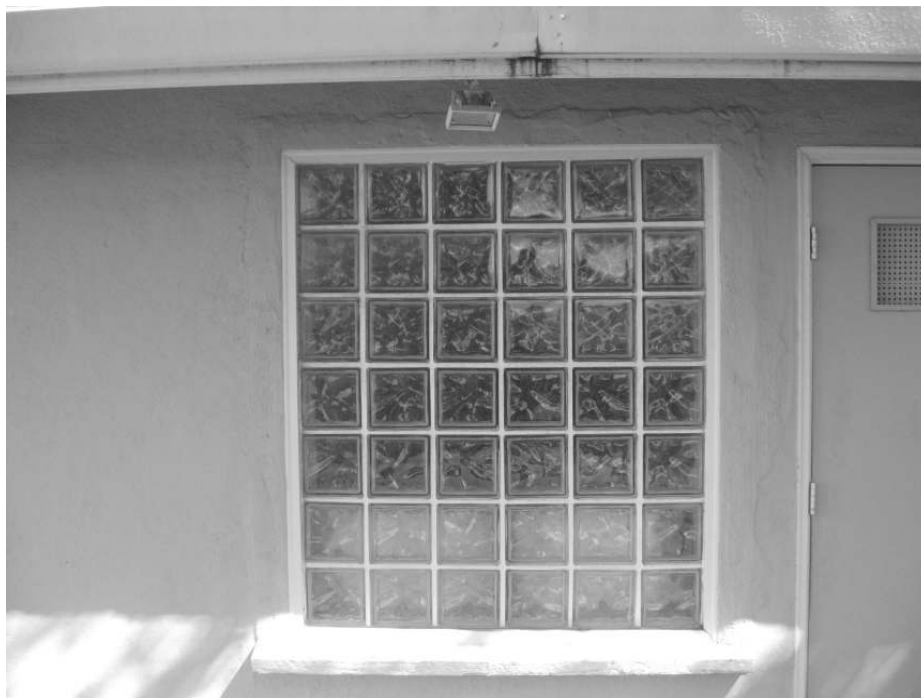
Photo 14: Detail of glass block window on southern facade.
