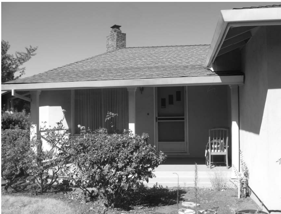
Photo 4: View of the entry and porch.
