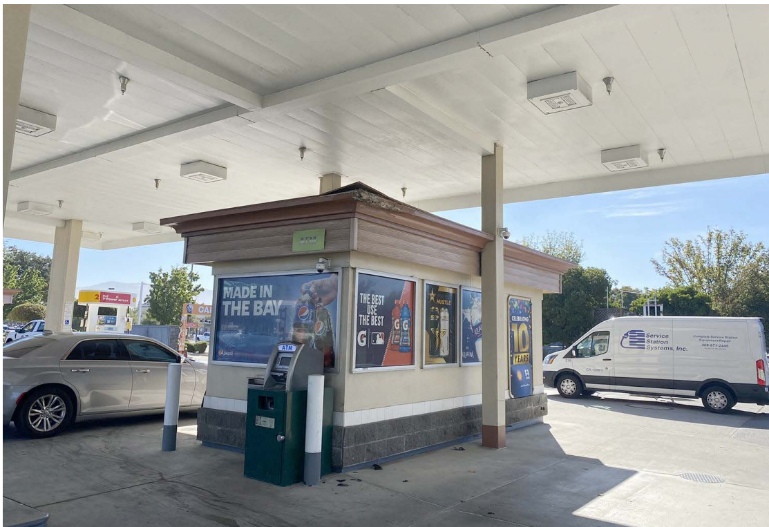
Photo No. 2 Fuel pump building
