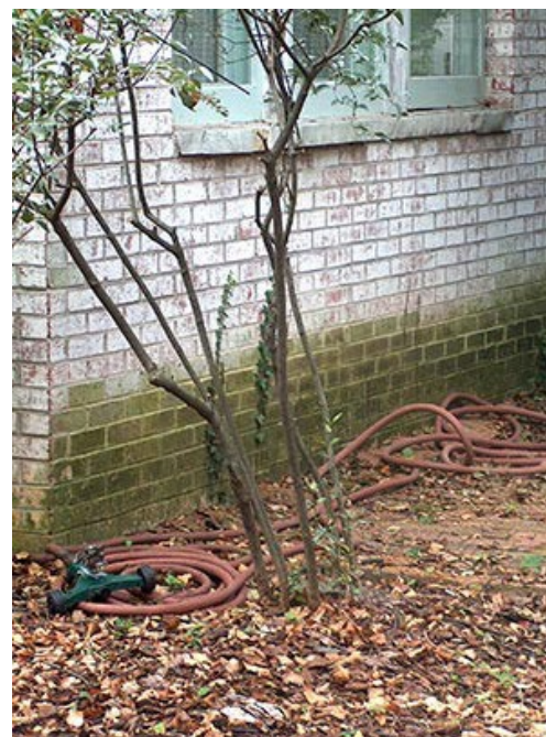
Figure 16. This chronically wet area has a mildew bloom brought on by heat generated from the air-conditioning condenser unit. The dampness could be caused by a clogged roof gutter, improper grading, or a leaking hose bibb.
