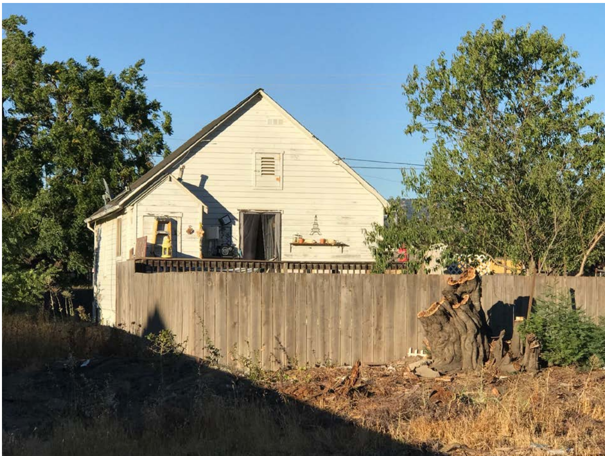
Photograph 4 18755 Old Monterey Road, Morgan Hill CA View: Rear (west) facade Small addition attached to the building on the left. Camera facing: East
