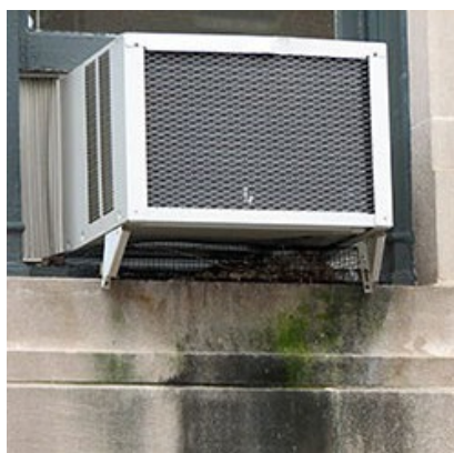
Figure 13. Window air conditioning units can cause damage to surfaces below when condensation drips in an uncontrolled manner. Drip extension tubes can sometimes be added to direct the discharge.
