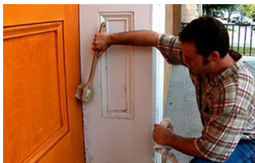
Figure 9. To help extend a repainting cycle, dirt and spider webs should be removed before permanent staining occurs. In this case, a natural bristle brush and a soft damp cloth are being used to remove insect debris and refresh the surface appearance.
