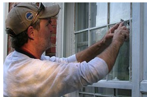
Figure 11. Glazing putty should be maintained in sound condition to prevent unwanted air infiltration and water damage. New glazing putty should be pulled tight to the glass and edge of the wood, creating a clean bevel that matches the historic glazing
