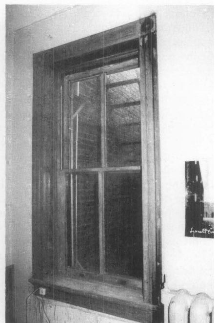
Figure 4f. Following the relatively simple repair the window is weathertight, like new in appearance, and serviceable for many years to come. Both the historic material and the detail and craftsmanship of this original window have been preserved. Photo: John H. Myers
