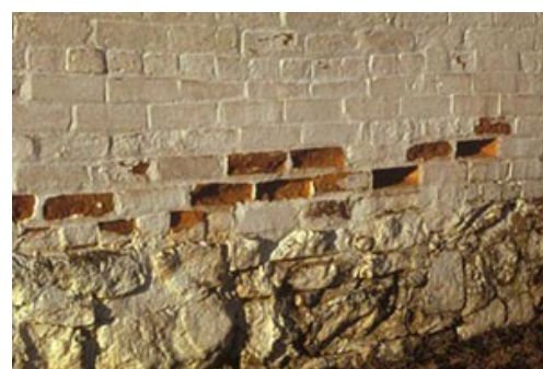
Figure 10. Repointing of masonry should usually be approached as repair rather than maintenance work in part because of the need for a skilled mason familiar with historic mortar. In this case, a moisture condition was not corrected and the use of a waterproof coating and off-the-shelf Portland cement mortar trapped water and resulted in further damage to these 19th century bricks. Photo: NPS files
