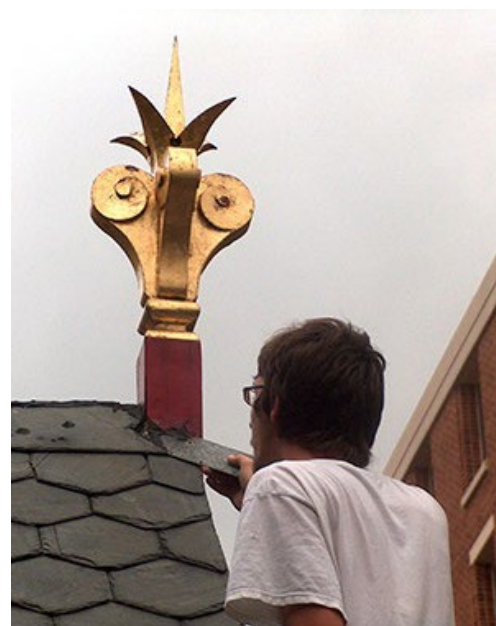
Figure 5. The use of a sealant to close an exposed joint is not always an effective long-term solution. Where this decorative wood element connects to the slate roof, the sealant has failed within a short time and a proper metal flashing collar is being fitted instead. Photo: Bryan Blundell.
