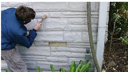
Figure 6. Stucco applied to an exterior wall or foundation was intended to function as a watertight surface. Unless maintained, rainwater will penetrate open joints and cracks that may occur over time. A spalled section of stucco indicates some damage has occurred and a wooden mallet is being used to tap the surface to determine whether the immediate stucco has lost adhesion. Photo: Bryan Blundell.
