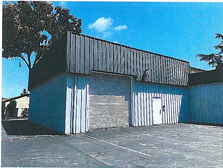
Unit 5 main entrance, showing warehouse entrance on left side and main entrance door to the right.
