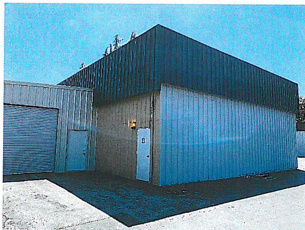
Back of building showing warehouse exit and adjoining storage unit (owned by Landlord and not part of unit 5)
