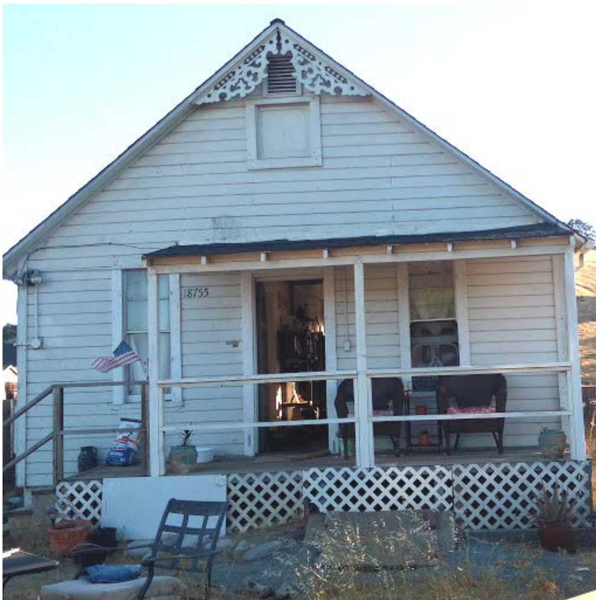
Photograph 1 18755 Old Monterey Road, Morgan Hill CA View: Front (east) facade
