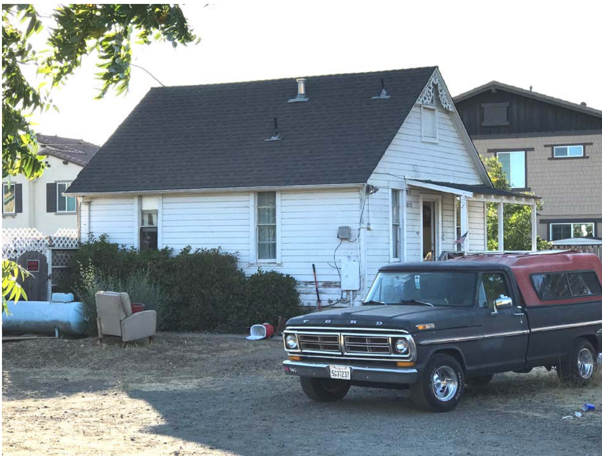
Photograph 2 18755 Old Monterey Road, Morgan Hill CA View: Front (east) and south side facade Camera facing: NW
