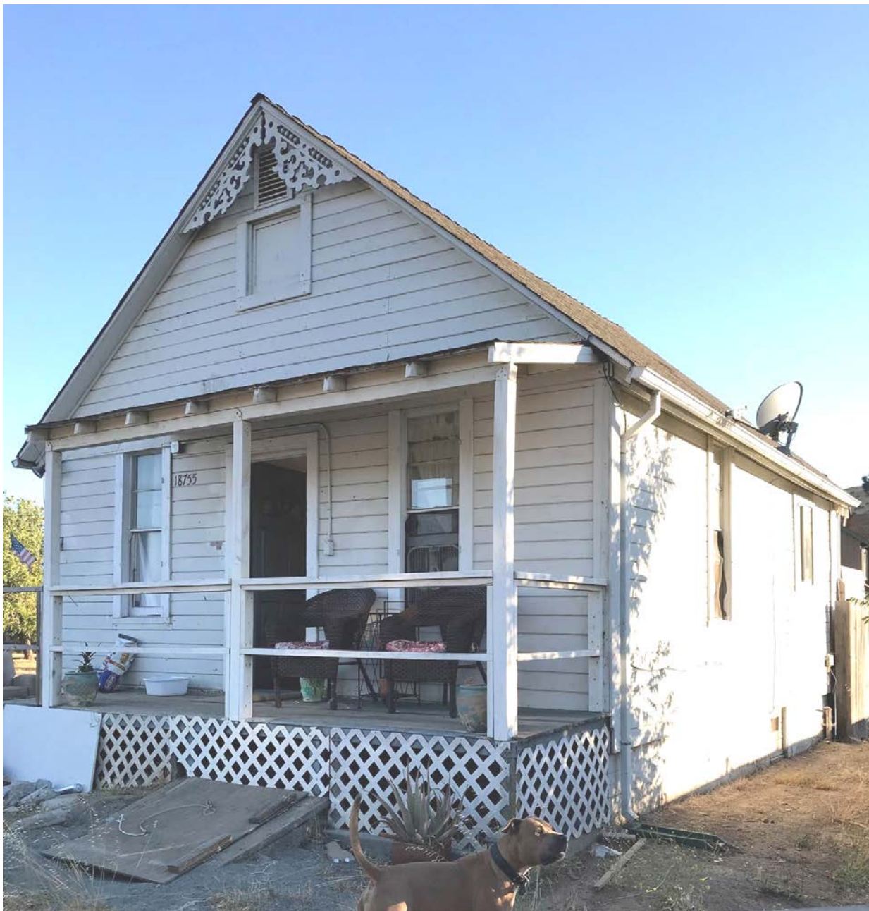
Photograph 3 18755 Old Monterey Road, Morgan Hill CA View: Front (east) and north side facade Camera facing: SW
